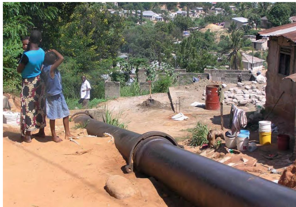
Water supply pipeline running directly through an urban slum in Dar Es Salaam, Tanzania.
